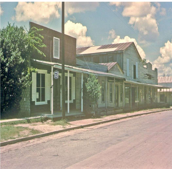
Picture taken in Mid-60's. on Main Street. First building on left is now the Nesting Company.
